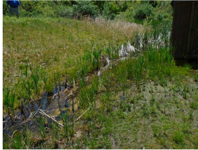
Photo 10: W side of adjacent property with drainage issues. Orientation: Southwest facing view
