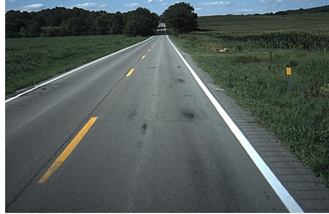
RUTTING = POOR
