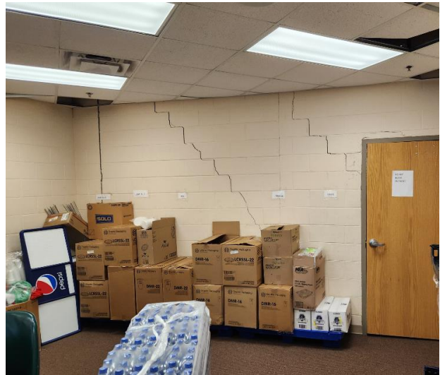
Photographs No. 5 and 6: Cracks in upper floor of stairwell and storage room.
