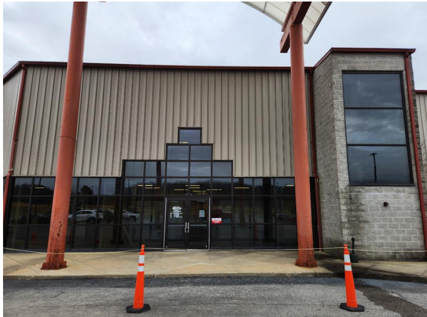
Photograph No. 4: Front View of the Sportsplex
