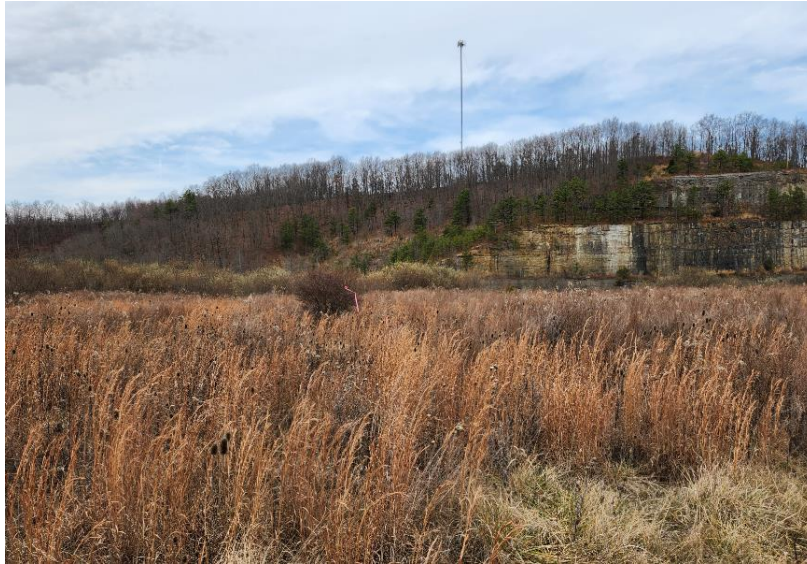
Photograph No. 1: View looking west toward boring B-1 (pink flag) and toward Highway 80. The cut is on the west side of highway 80.
