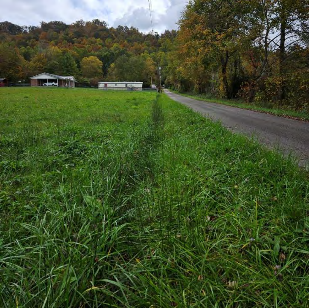
Figure 4-1. View of the ditch within Twin Meadows APE adjacent and parallel to Twin Meadows Road, Booneville, Owsley County, Kentucky. From northwest corner of APE facing south-southeast.
