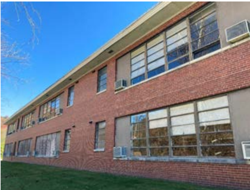
West side of building.
