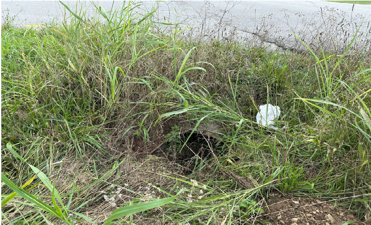
Photo 16 Comments: Representative stormwater culvert on subject property.
